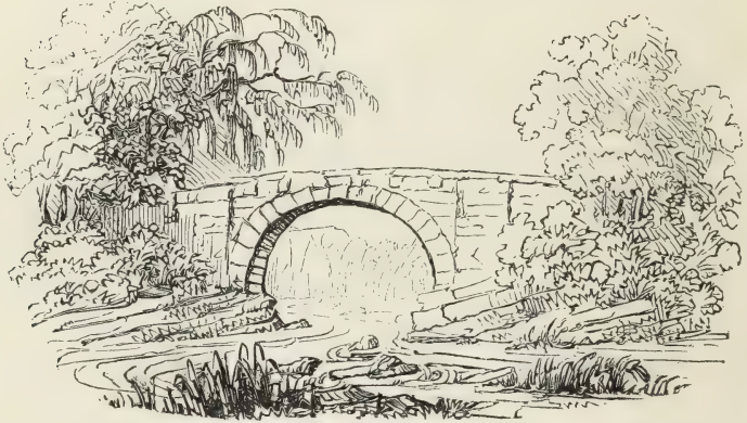
[Fig. 57. Bridge in the grounds of Harewood Hall, shewing the artificial disposition of masses of stone in imitation of ledges of rock in the bed of the river.]
